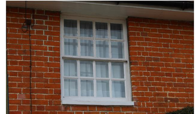
Figure 30 Example of a timber sash window
